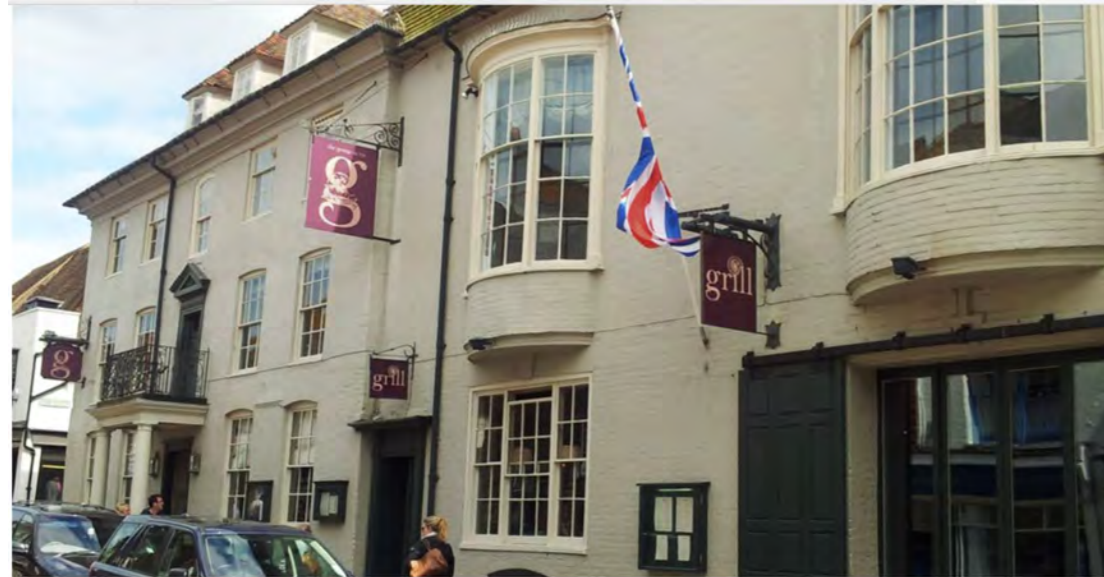
Fig 16 – Pre-fire. C.2016 with the two light green tones to the elevations, dark green to the doors, surrounds and plinths, windows frames etc cream
