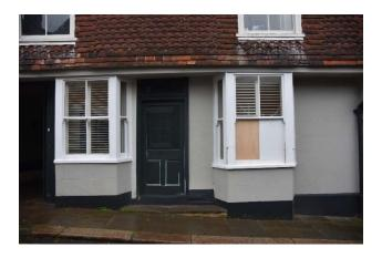
Only twentieth-century paints were found in samples taken from the rendered walls, but in one sample from the side of the door architrave we can see layers of limewash sandwiched between layers of oil paint used for the door, and the facade of this part of the building must have been limewashed through the nineteenth century.
